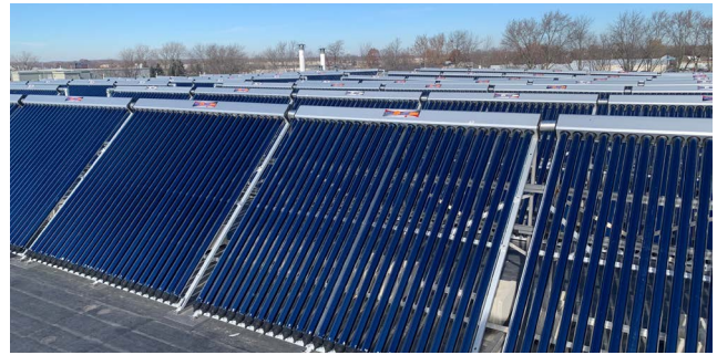
Close up of SunQuest 250 solar thermal collectors
