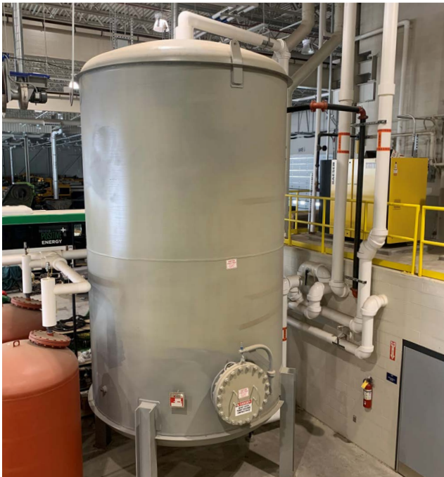
10,000-gallon hot water storage tank preheated by the solar thermal array
